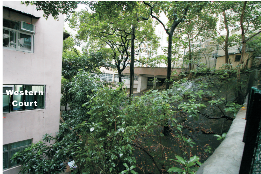
LR4.2 Manmade Slope next to Western Court
